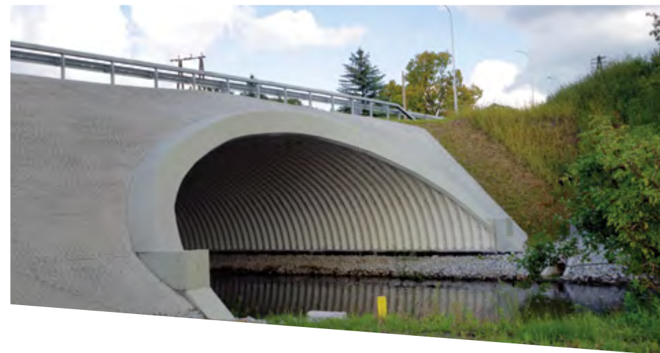
Arch bridge with concrete collar, Poland
