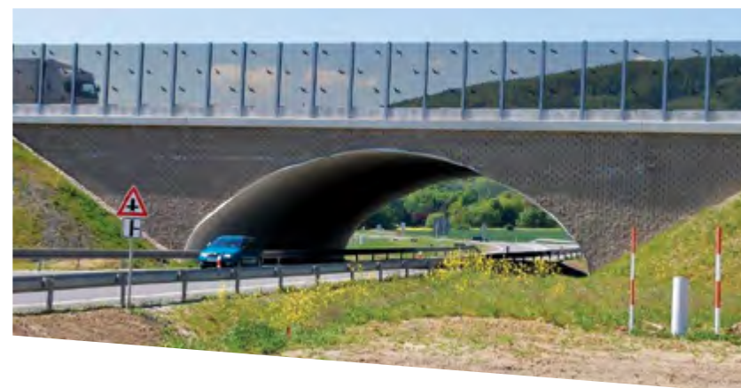
Grade separation with blocks facing (MSE walls), Czech Republic
