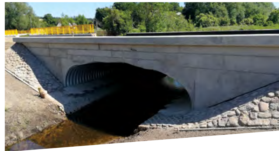
Bridge with concrete paving, Poland
