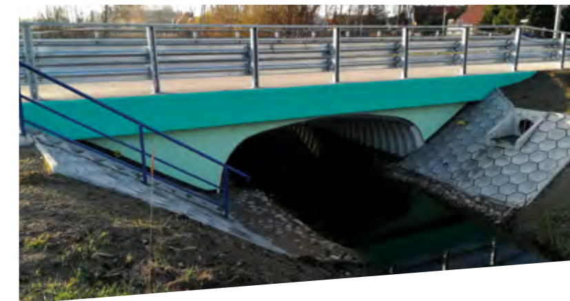
Bridge with concrete block facing, Poland
