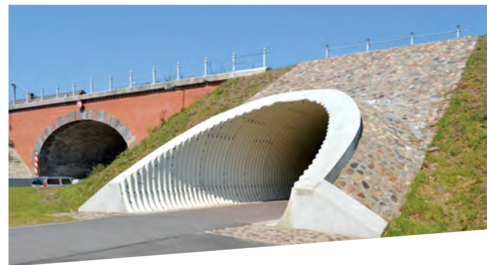
Underpass under the railway line, Latvia
