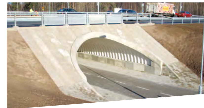
Grade separation with concrete paving, Finland
