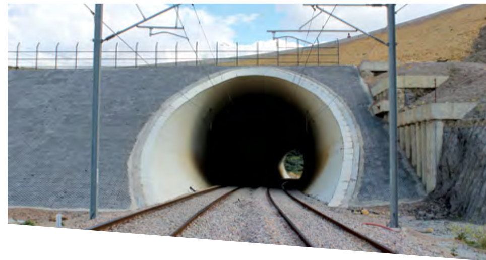
Railway tunnel, Algeria
