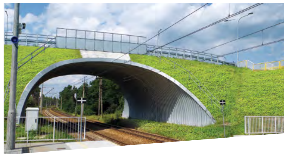
Grade separation over railway line, Poland
