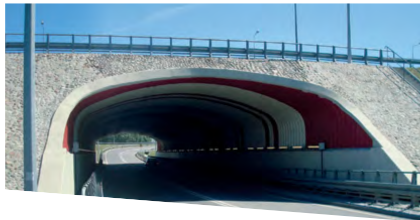
Grade separation, Poland
