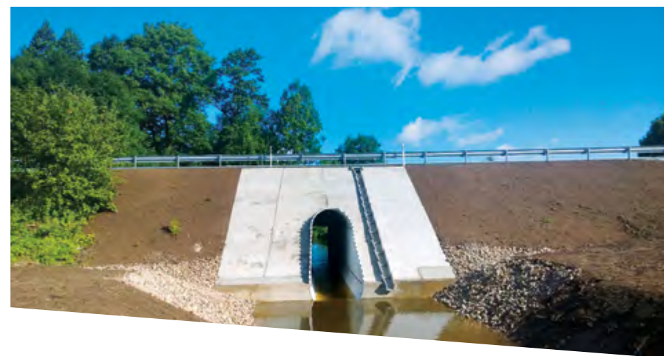
Culvert with concrete paving, Lithuania
