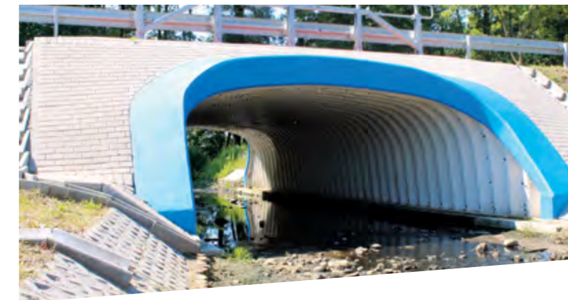
Bridge with concrete block facing, Poland
