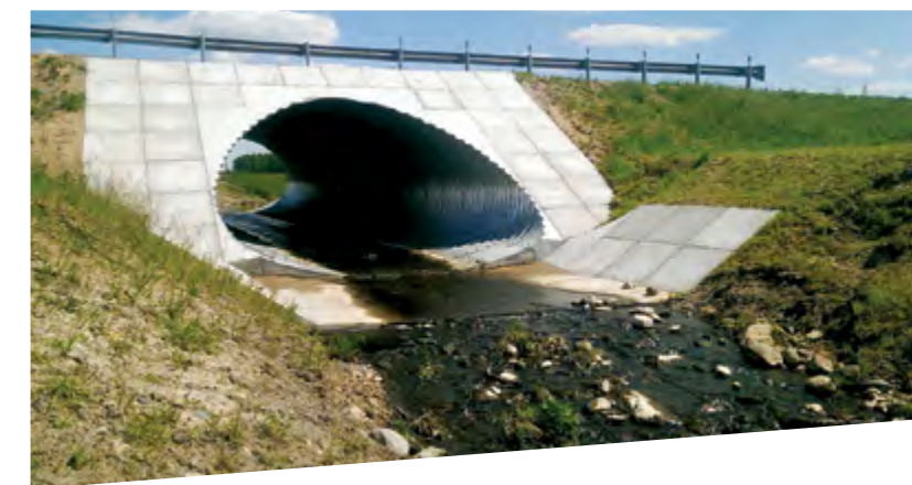
Bridge over Turya river, Belarus
