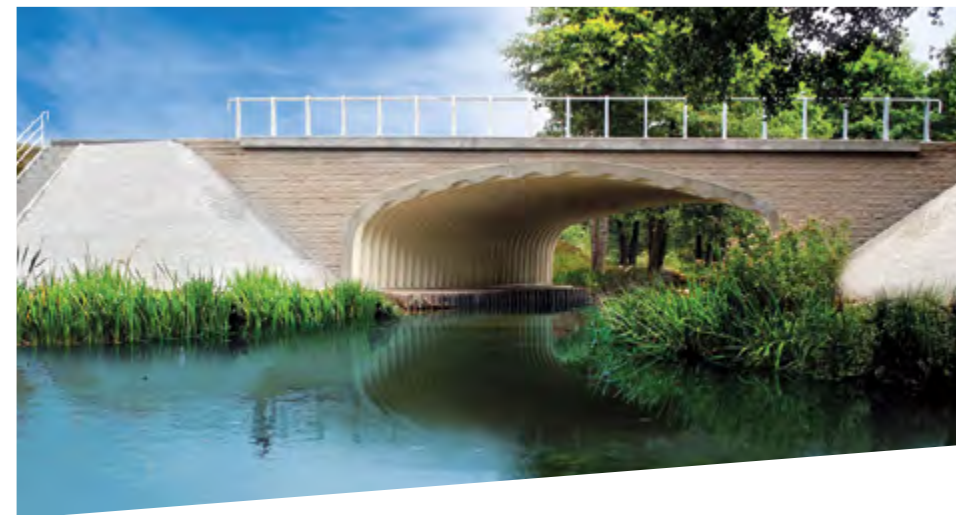
Bridge over Rospuda river, Poland
