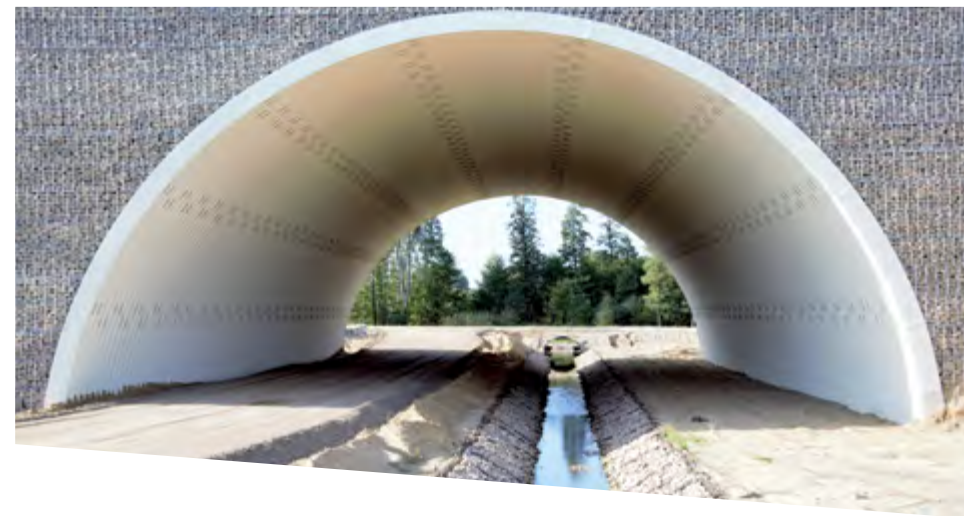
Bridge with wire mesh finish (MSE walls), Poland
