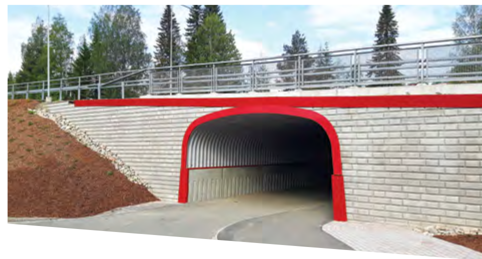
Underpass bridge in Kuopio, Finland
