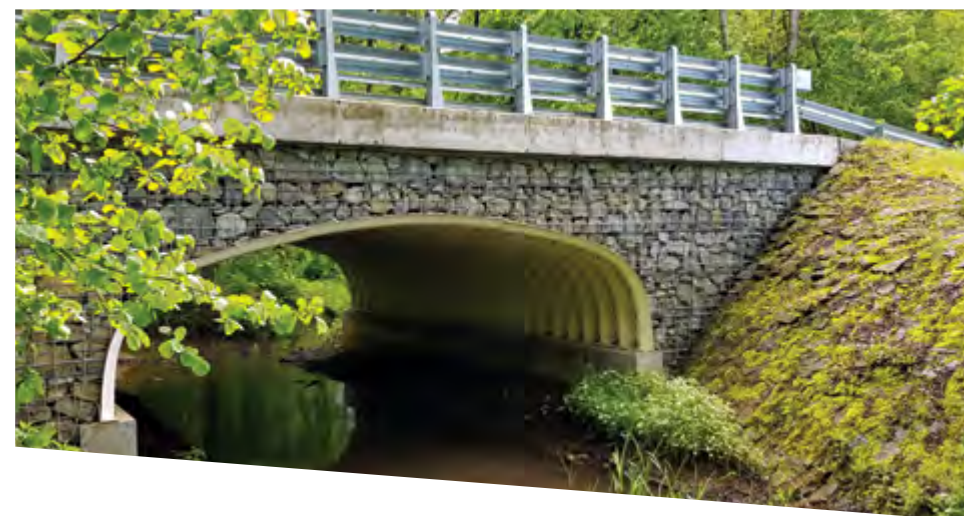
Bridge with wire mesh finish, Poland
