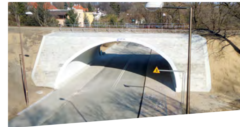
Grade separation under railway, Poland
