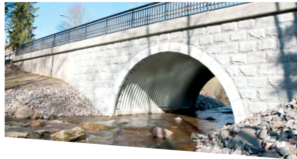
Bridge with blocks facing, Finland
