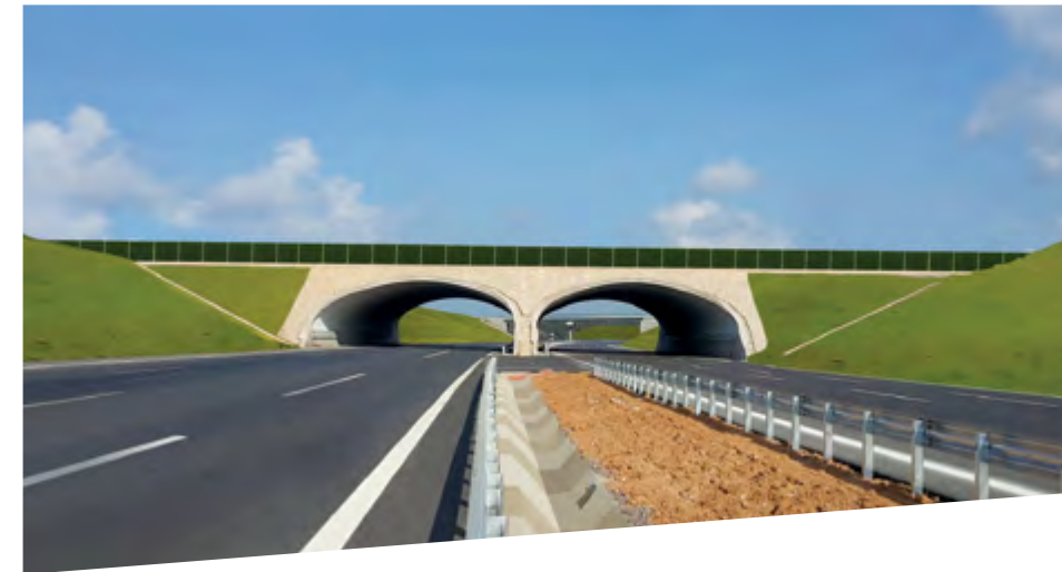
Animal overpass with beveled ends, Turkey
