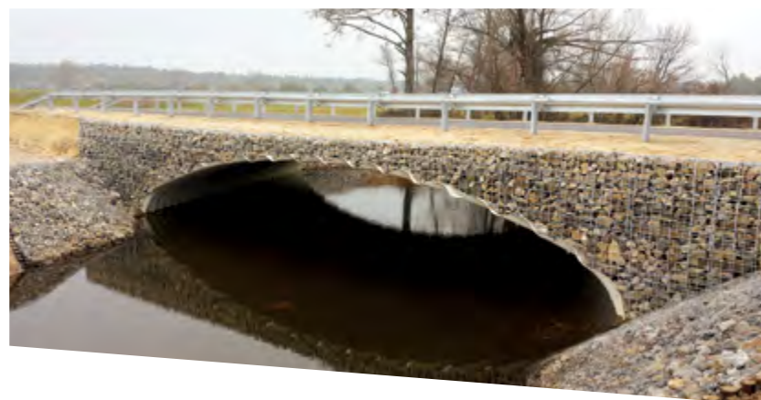
Bridge with wire mesh wall, Poland
