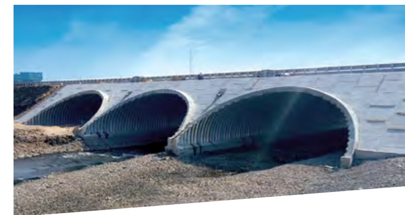
Bridge over Lebeda river, Belarus
