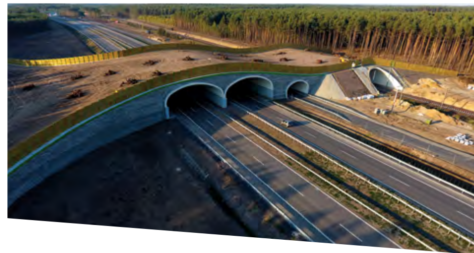
Animal overpass, S5 road in Poland
