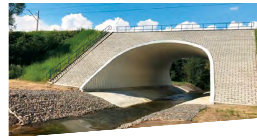
Railway bridge, Poland
