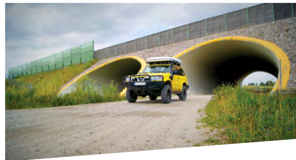
Underpass under national road, Poland
