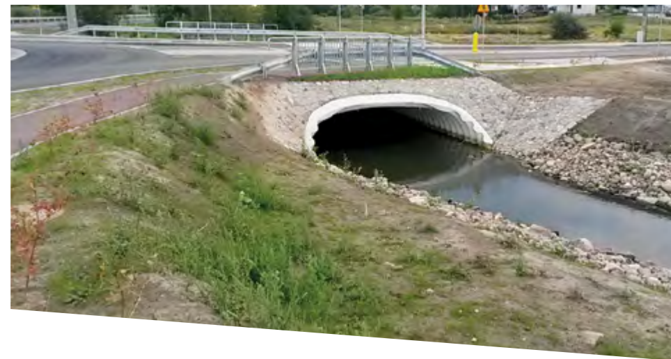
Bridge with natural stone facing, Poland
