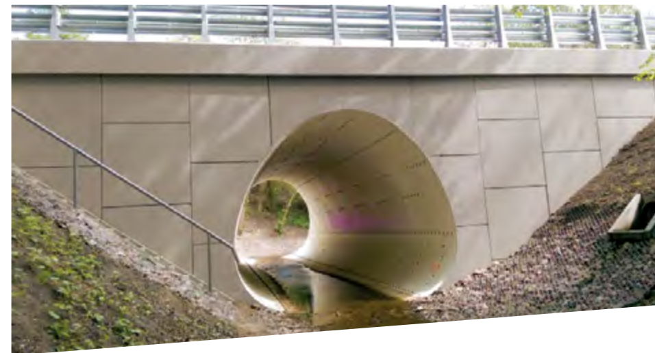
Bridge with panel facing, Poland
