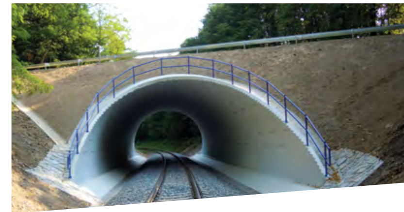
Grade separation over railway line, Bolatice, Czech Rep.
