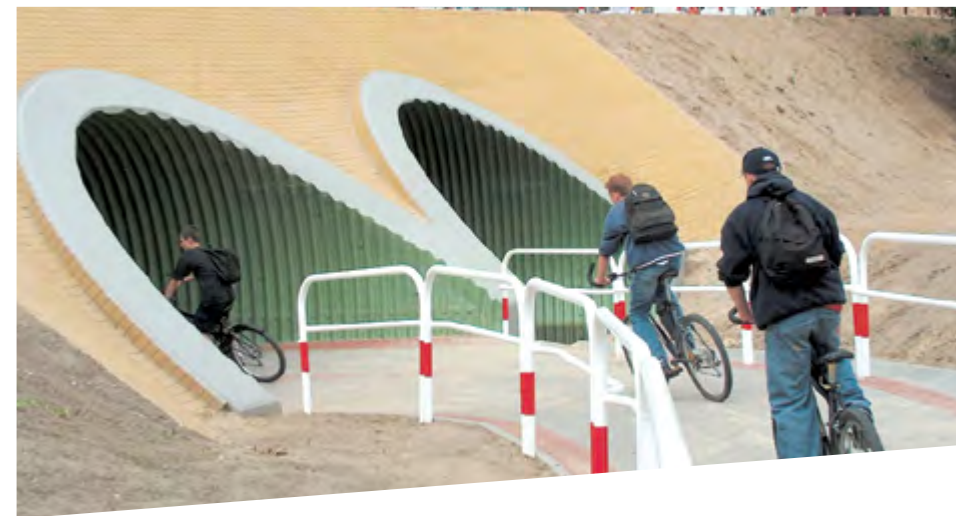
Pedestrian underpass and bridge, Poland
