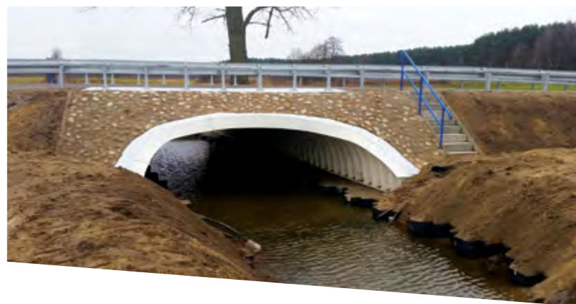
Bridge with stone facing, Poland
