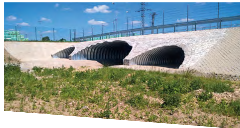
Three-span bridge, Poland
