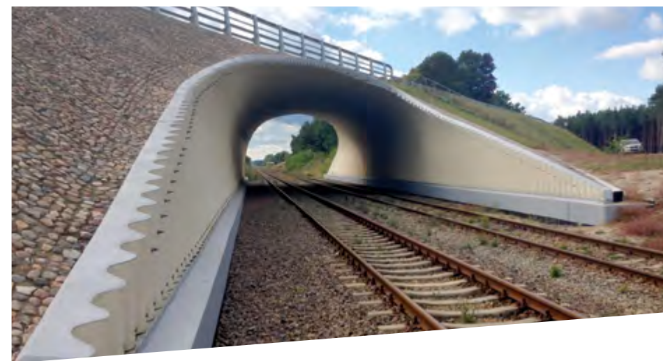
Grade separation over railway line, Poland
