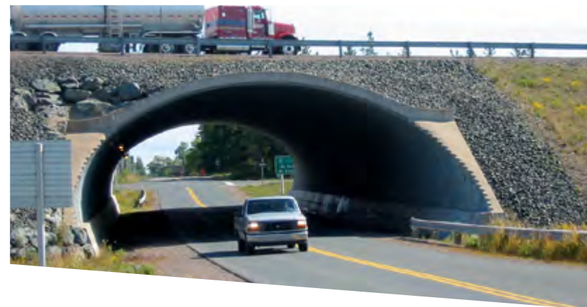
Grade separation, Canada
