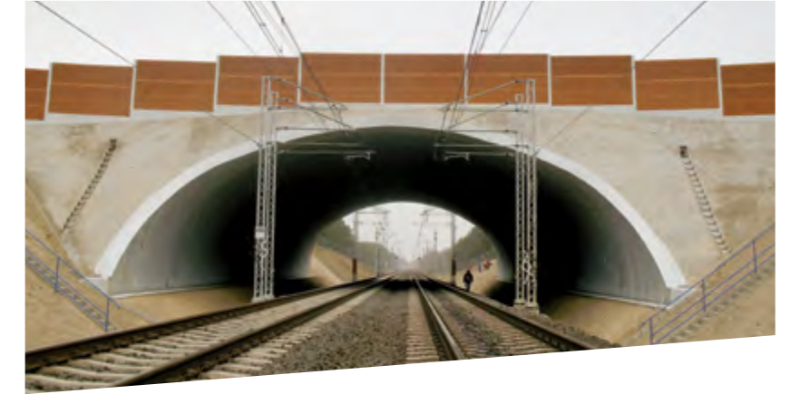
Animal overpass over railway line, Poland
