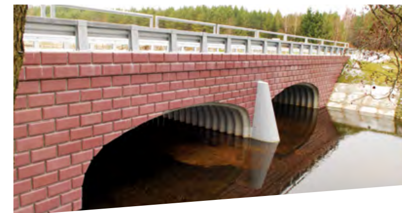
Bridge with red block headwall, Lithuania
