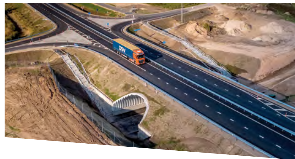
Underpass under national road, Lithuania
