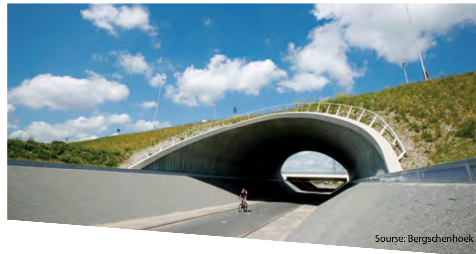
Grade separation, Netherlands
