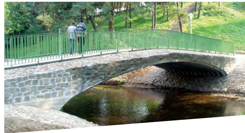
Pedestrian foot bridge, Poland
