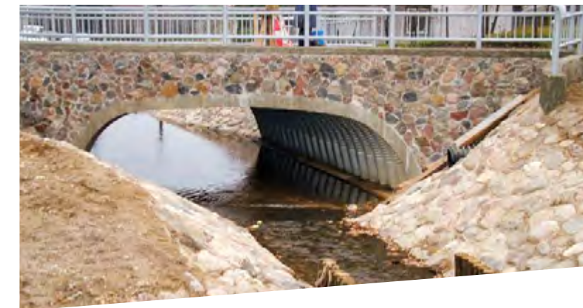
Pedestrian foot bridge, Lithuania
