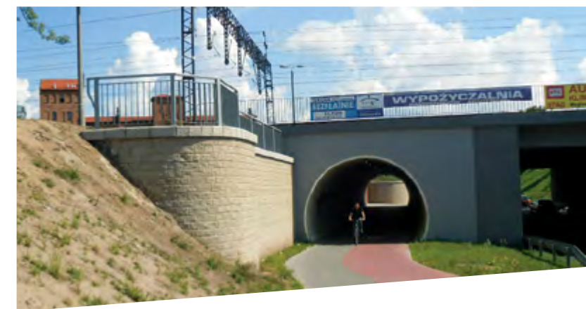
Railway bridge, Poland
