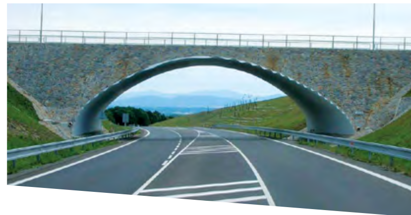
Grade separation with block paving, Bilov, Czech Republic
