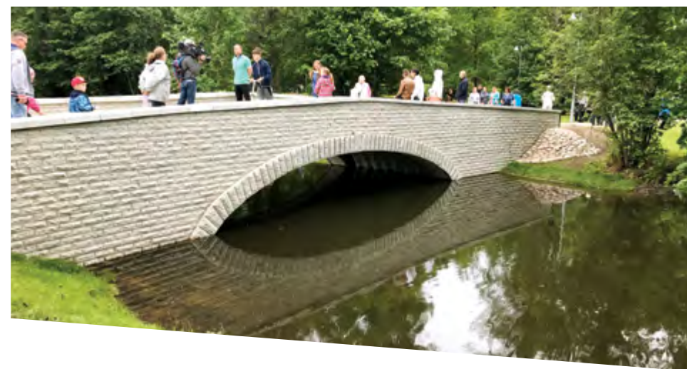
Pedestrian foot bridge, Estonia
