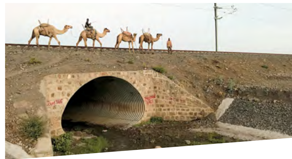
Culverts under the railway line, Ethiopia
