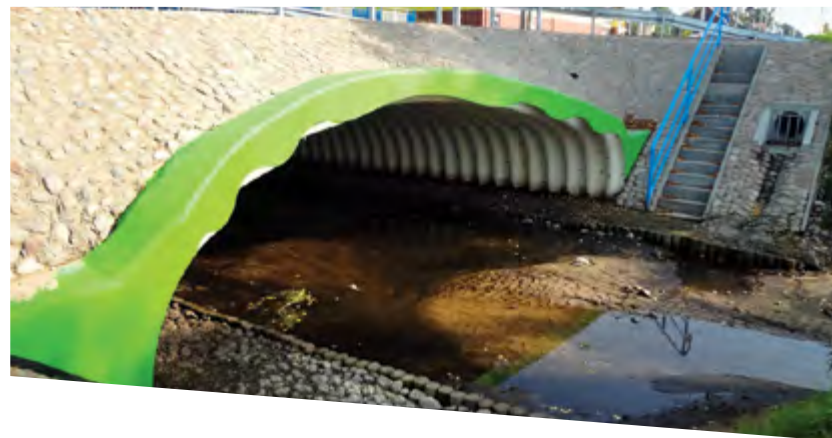
Bridge with natural stone facing, Poland
