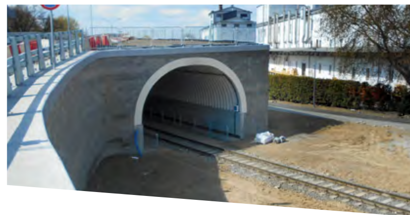
Grade separation over railway line, Poland
