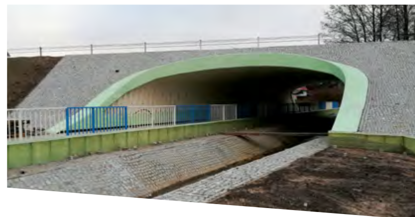
Bridge with stone paving, Poland
