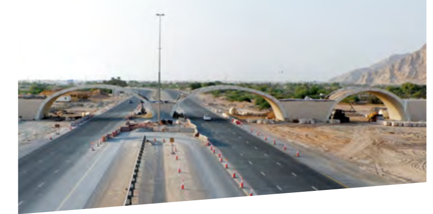
Backfilling process in progress.
