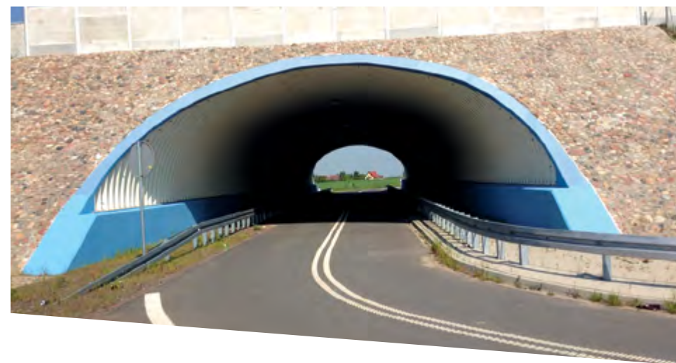
Grade separation, Poland
