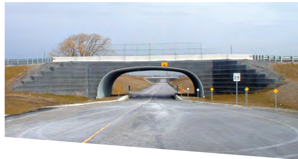
Grade separation under railway with MSE walls, Canada
