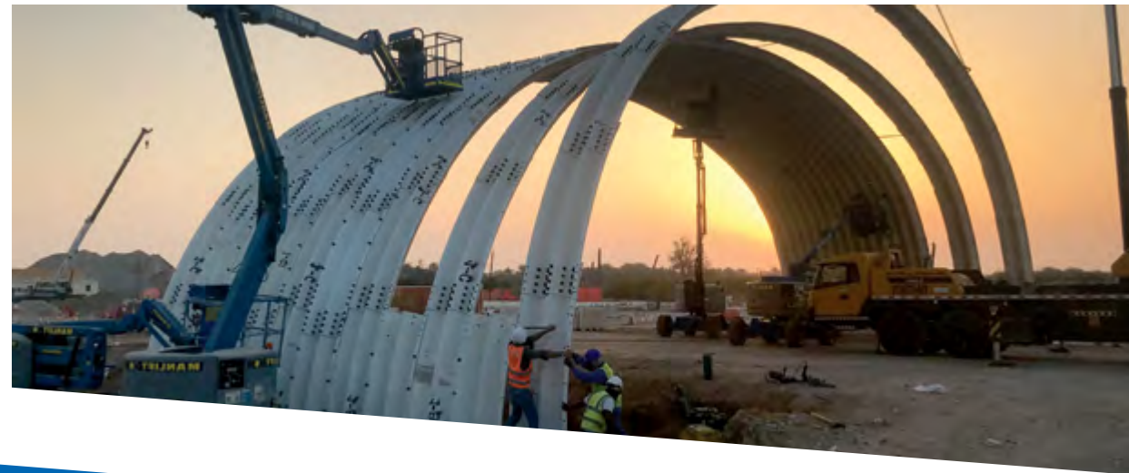
First UltraCor rings erected.
