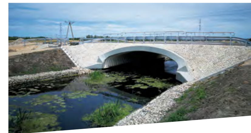
Bridge with stone paving, Poland
