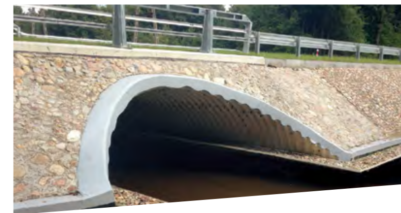
Bridge with natural stone facing, Poland
