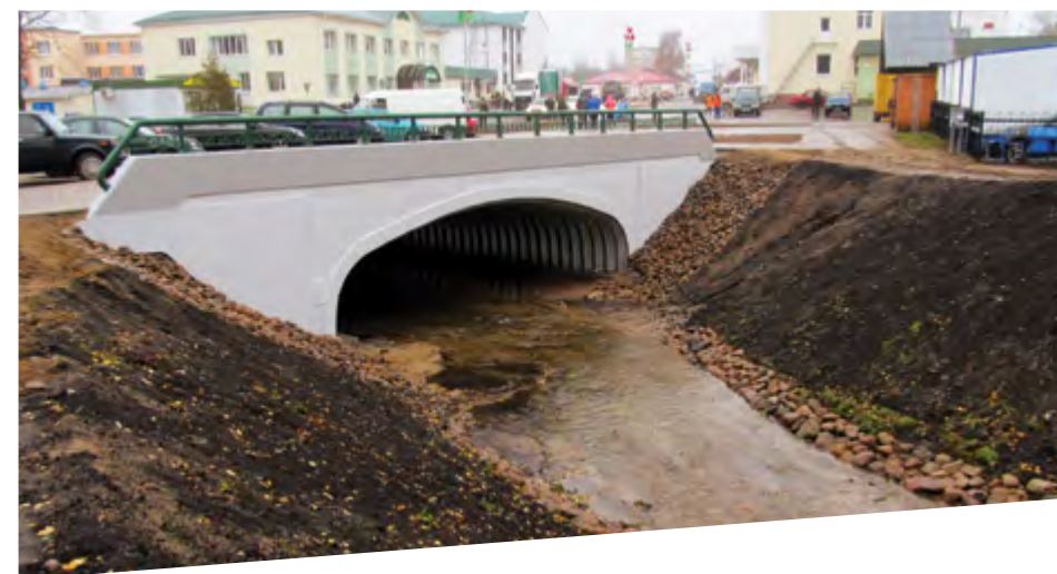
Bridge over Dyatlovka river, Belarus
