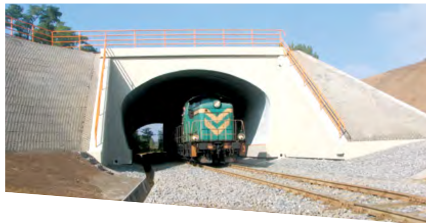
Grade separation over railway, Poland
