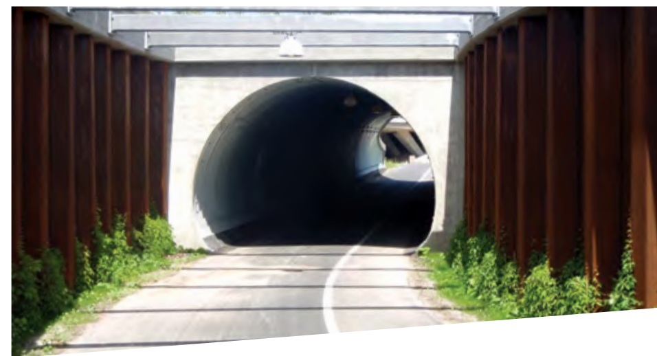
Cycleway underpass, Denmark
