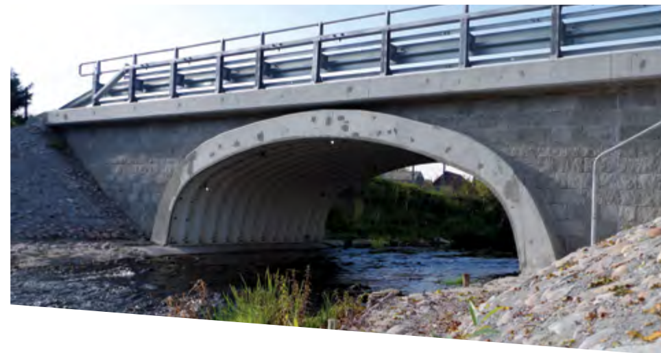
Bridge with MSE walls finish
