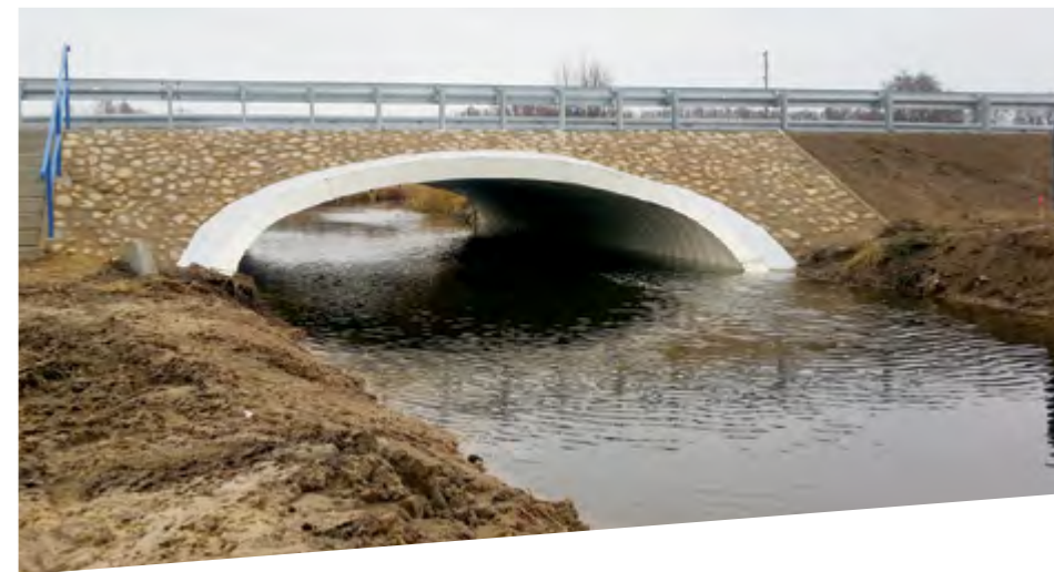
Bridge with stone facing, Poland
