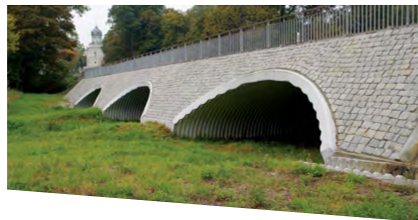
Three span bridge, Poland
