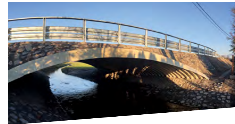
Bridge with stone facing, Poland
