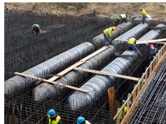
Trenchcoat™ film can be applied on either one or both sides of the pipe.
