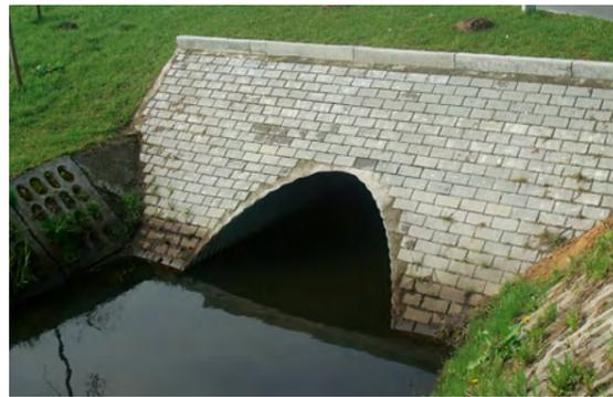
For the same water level the pipe-arch shape has 65%-100% more water flow capacity than a round pipe with the same rise.
