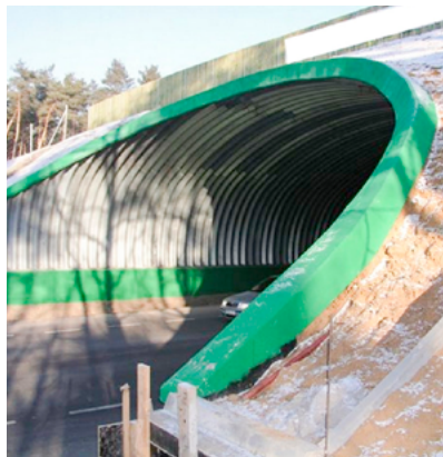
concrete headwall – beveled end.
